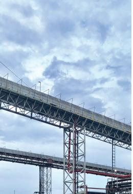
Controlling dust from bagasse storage areas such as using the water spray to prevent diffusion of bagasse and installing the cover of the bagasse conveyor bridge.
